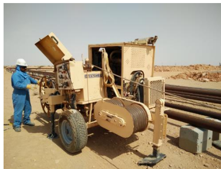
Gambar II.2. Pulling Machine. (dokumentasi pribadi; Oman,2016)
