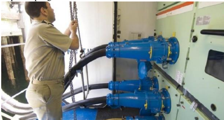
Gambar 2.6 Shore Power Connection Box sumber: abb.com
