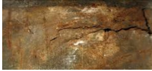
Gambar 2. 4 Korosi Sumuran ( Scribd.com/korosi )
