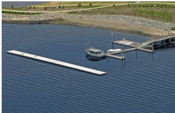
**Gambar 2. 1** *Pontoon Floating Breakwater*
