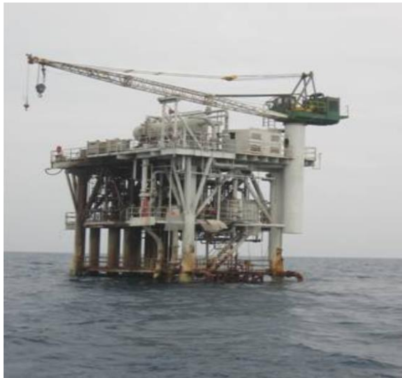
Gambar 3.2. Platform LB (PT. Depriwangga Engineering)
