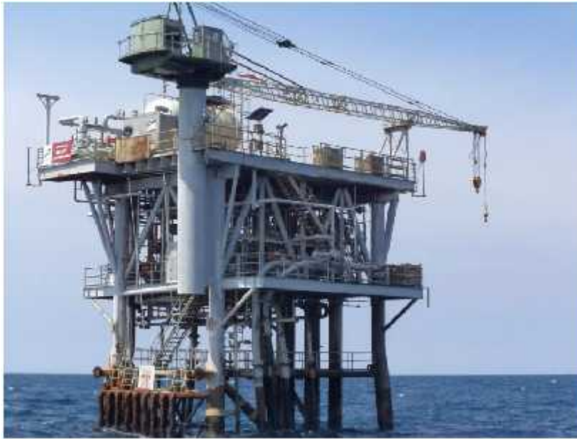
Gambar 3.2 UA Well Platform PHE ONWJ (PT.Tripatra Engineering)
