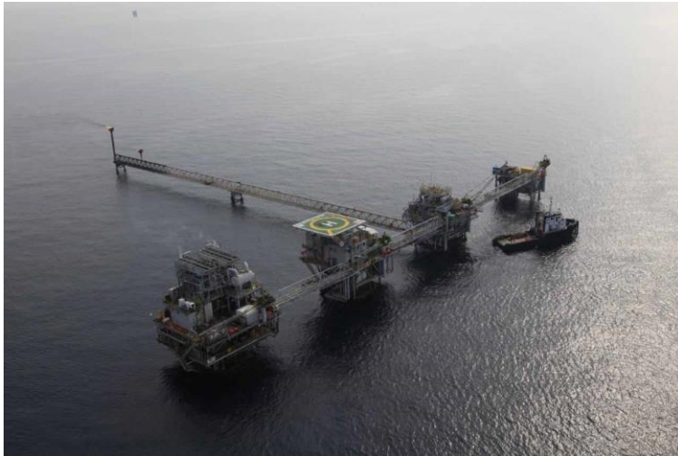
Figure 13 LIMA Flowstation Complex
