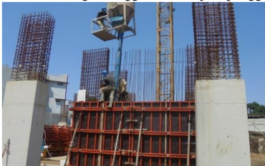
Gambar 6. 9 Pengecoran Shearwall
