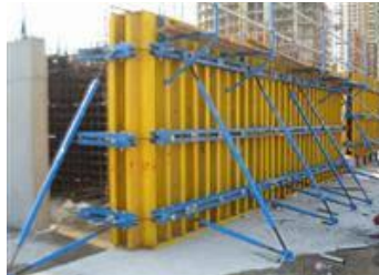
Gambar 6. 8 Bekisting Shearwall
