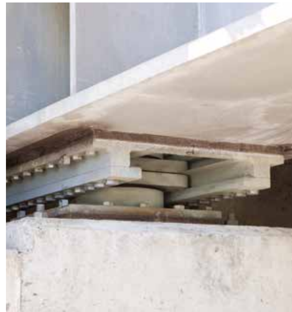
Dominion Bridge – Lévis, QC
