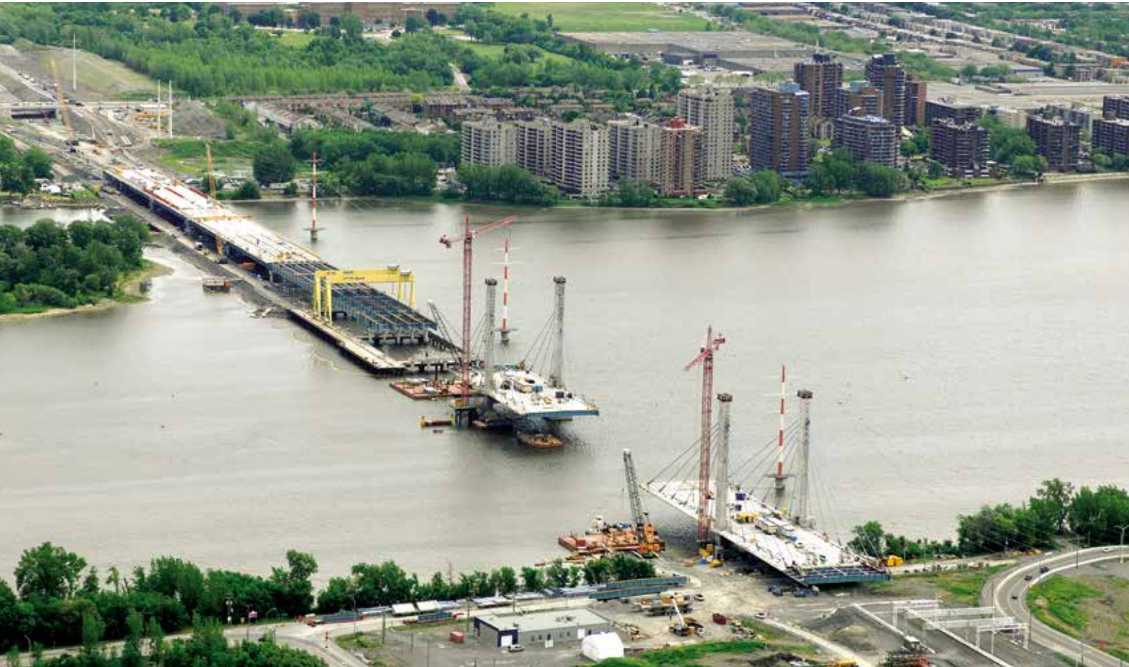
Highway 25 Bridge – Montreal/Laval, QC
