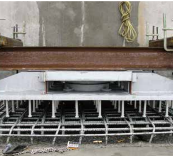
PM Series multidirectional bearing installed at pylon No. 11 of the Highway 25 Bridge.
