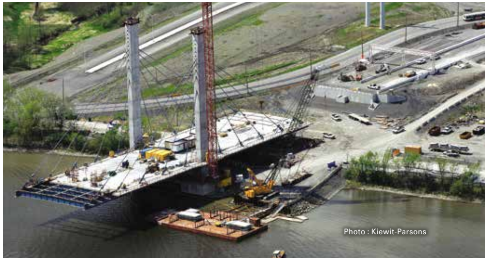
Goodco Z-Tech manufactured pot bearings and lateral restraint systems for the cable-stayed span of the new Highway 25 Bridge over the Rivière des Prairies.
