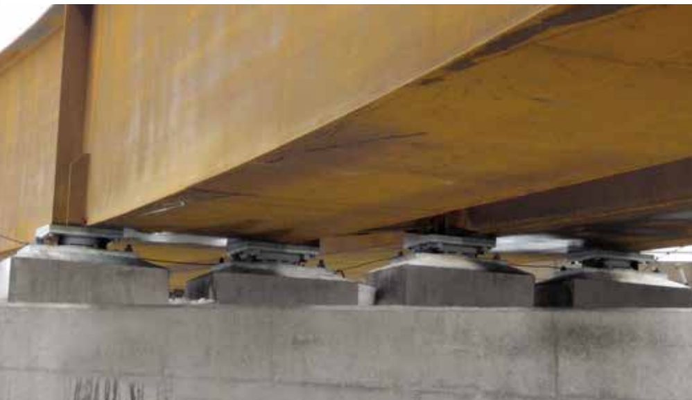
PMG Series unidirectional bearings (two in center) and PM Series multidirectional bearings (two on the sides) used under curved box girders.
