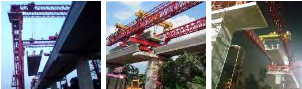
Gambar 2.2 Proses Erection dan Pemasangan U-Shape Girder (PT. Adhi, 2016)
