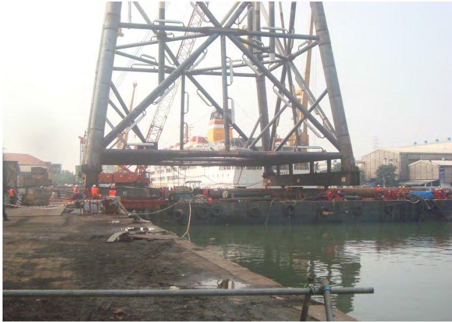
Gambar II.7 Proses Load Out Jacket (Sumber : PT. PAL Indonesia)
