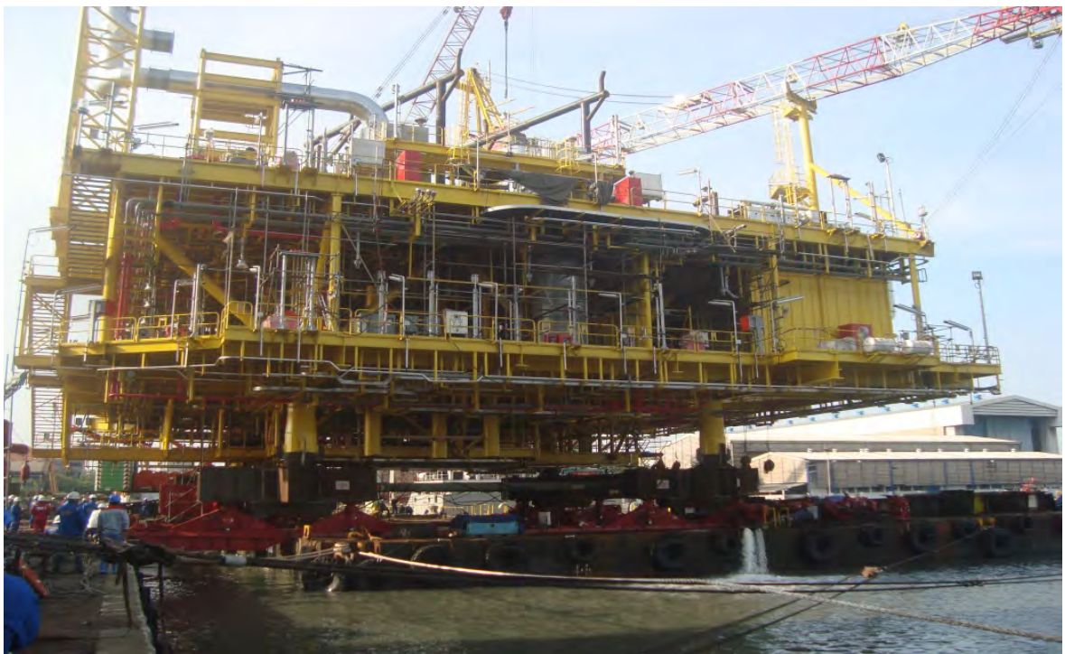
Gambar II.6 Proses Load Out Topside ke Barge (Sumber : PT.PAL Indonesia)
