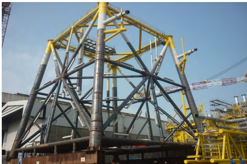
Gambar II.3 Jacket Structure (Sumber : PT.PAL Indonesia)
