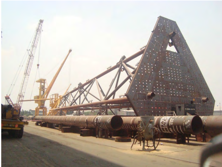
Gambar II.4 Proses Fabrikasi Jacket (Sumber : PT.PAL Indonesia)
