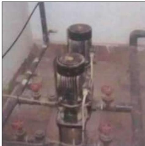
Gambar 4.21 Pompa *Booster* (PDAM, 2017)
