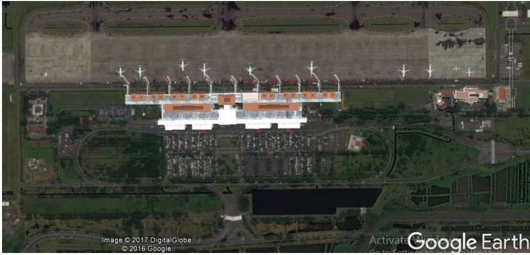
Gambar 1.5 Bandara Internasional Juanda, Surabaya (sumber: google earth)
