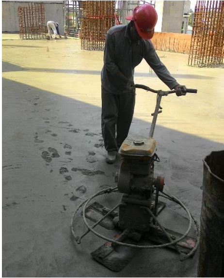
Gambar 4. 53 Proses Perataan Adonan Beton
