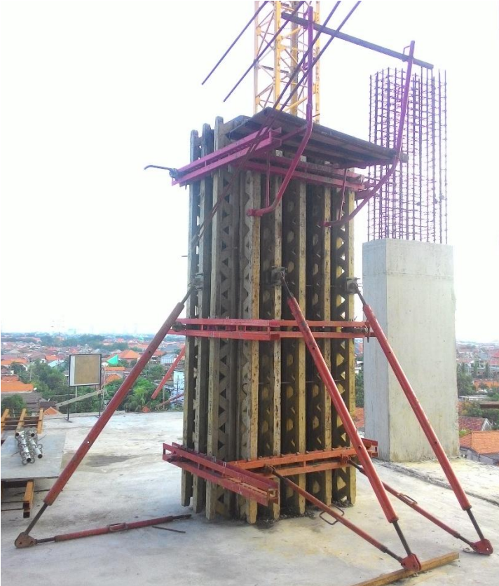
Gambar 4. 38 Posisi Form Work Lapangan
