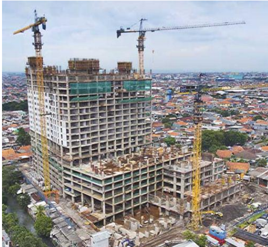
Gambar 4. 5 Posisi Tower Crane Gunawangsa Tidar Apartment
