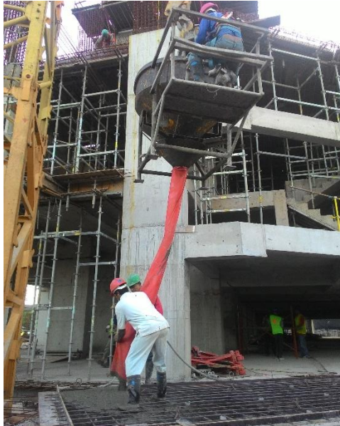
Gambar 4. 45 Proses Pengecoran Half-slab Lapangan
