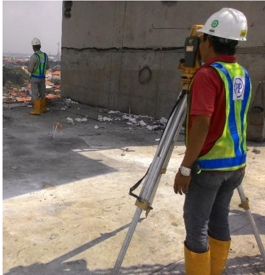
Gambar 4. 31 Proses Marking Lapangan
