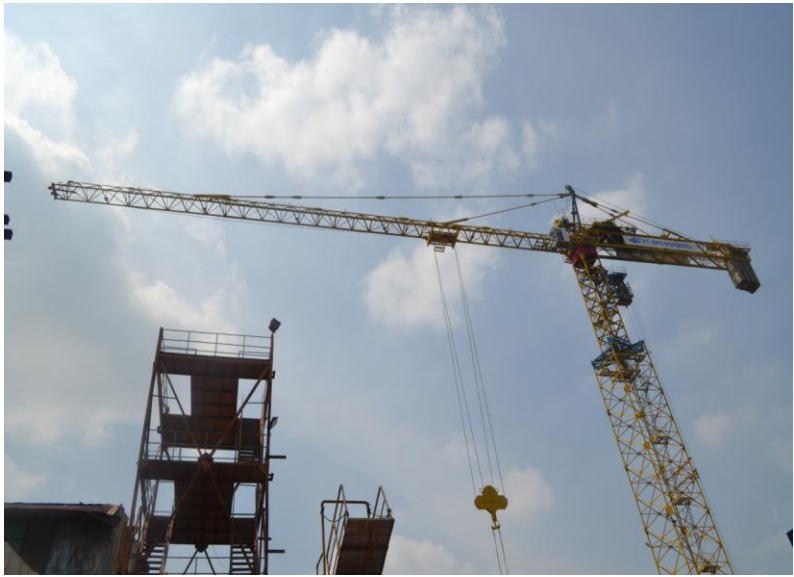
Gambar 4.1 Tower Crane Potain MD 900
