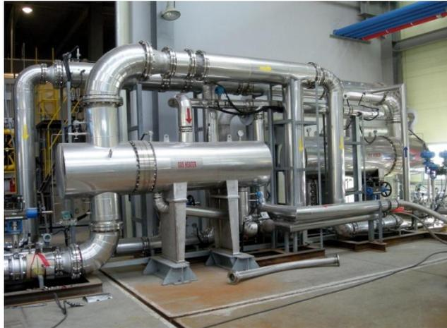
Gambar 5.26. LNG Vaporizer
