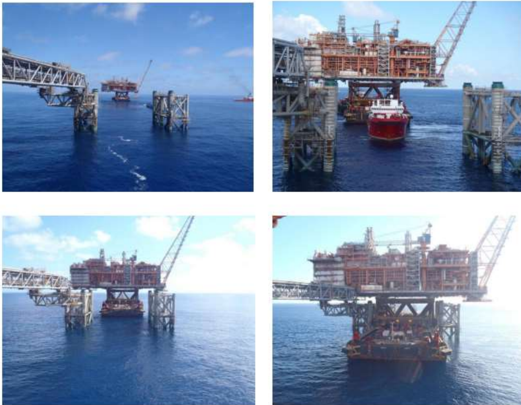
Gambar 2.2 Floatover Installation
