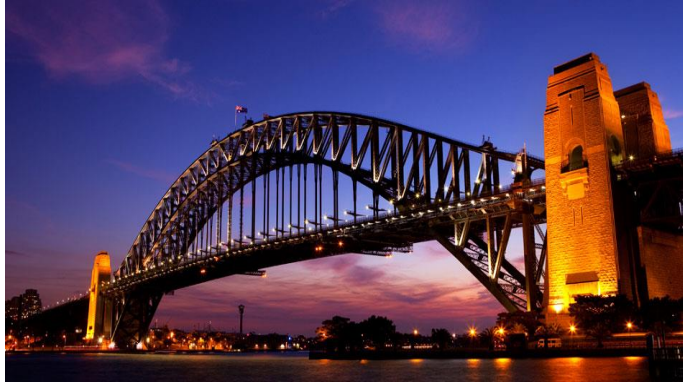
Gambar 2.3 Contoh a half – through arch Sydney Harbour di Australia
