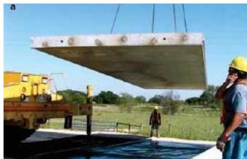
**Gambar 2. 3 Solid Flat Slab**
