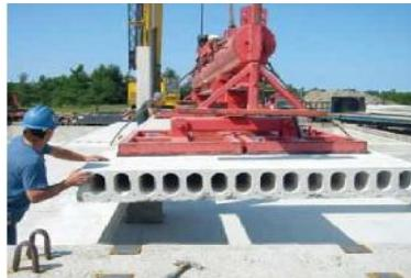
**Gambar 2. 2 Hollow Core Slabs**
