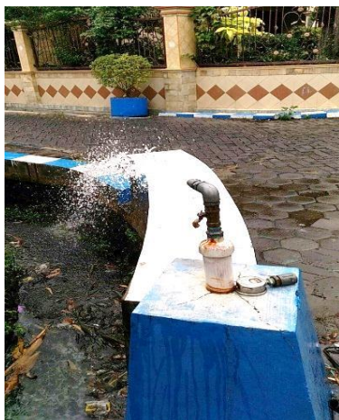
Gambar 4. 26 Proses Flushing
