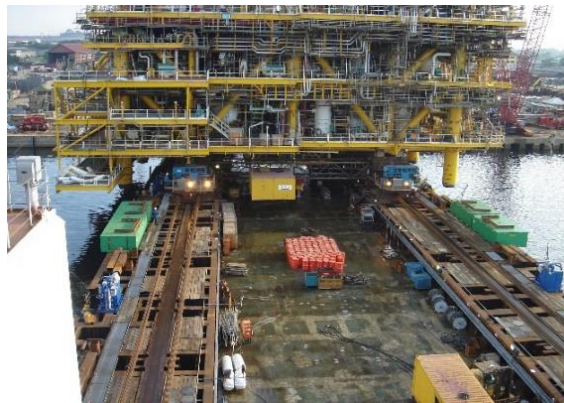
Gambar 2.4 Skidding System (Sumber: www.hmc.nl )
