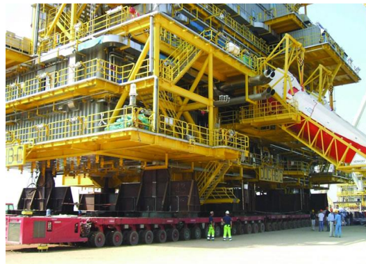
Gambar 2.5 Deck Struktur diatas SPMT (Sumber: www.fagioli.it )
