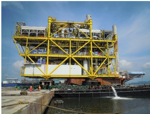
Gambar 2. 3 Loadout Metode Dolly ( www.heavyliftspecialist.com )
