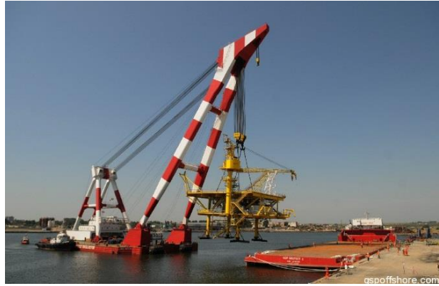
Gambar 2. 4 Loadout Metode Lifting ( www.gspoffshore.com )
