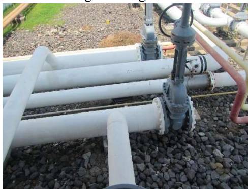
Gambar 3.4 Pipeline jalur buntu
