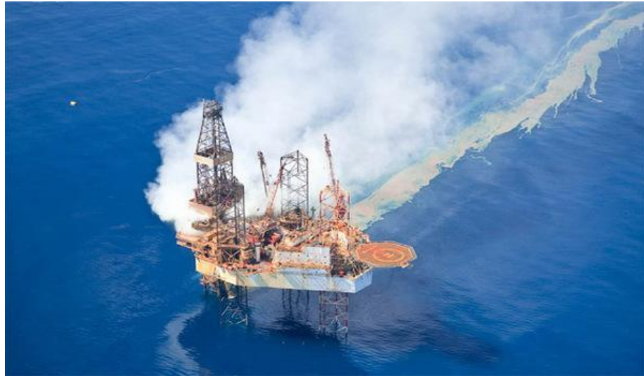
Gambar 1 Montara Wellhead Platform saat Meledak (Mengkaka, 2017)
