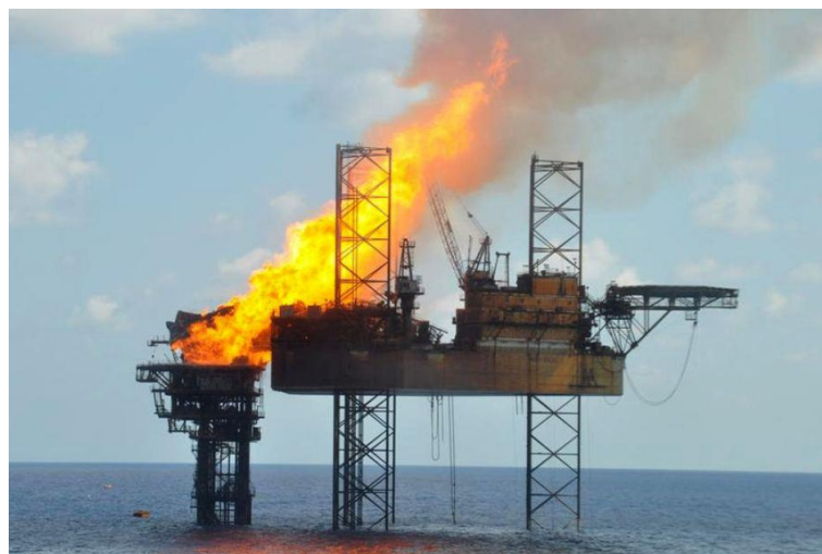
Gambar 13 Montara Wellhead Platform saat Terbakar (Lannin, 2016)
