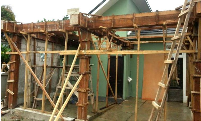
Gambar 2. 1 Bekisting Konvensional (Sumber : Ifadah Amalia, 2016 )
