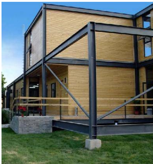
Gambar 4.18. Struktur Baja Expose Luar (Sumber : https://mybktouch.com/prefab-wooden-houses/ )
