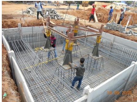
Gambar 4.18 : Contoh proses penanaman fine angle dan base section
