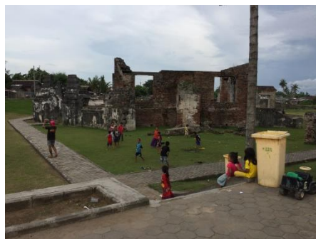
Gambar 4. 3 Istana Keraton Kaibon Sumber: Survey Primer, 2018
