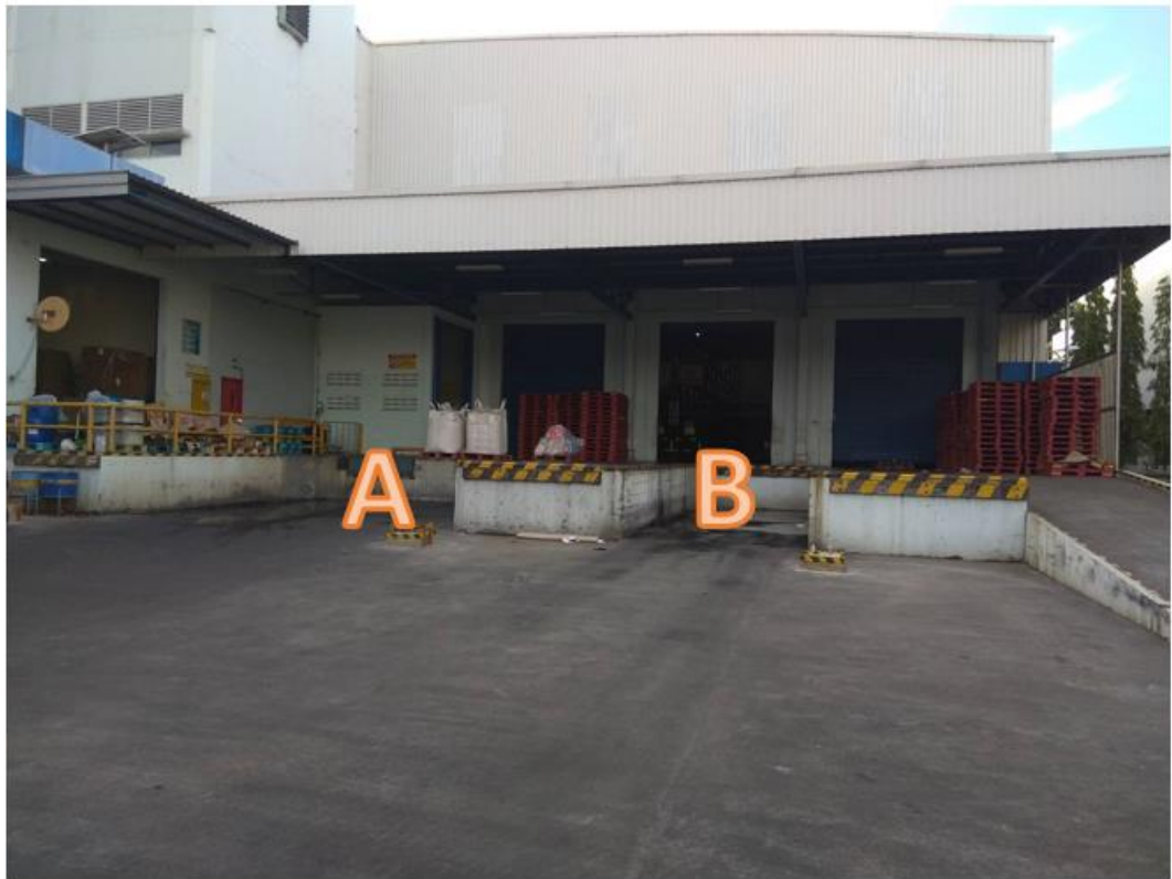
Figure 5.5 Two Loading Unloading Dock.
