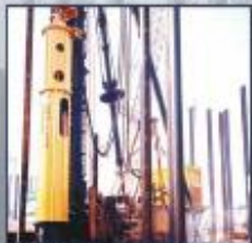
SGH-2015 20ton RAM WEIGHT with 1.5m STROKE
