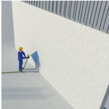
Gambar 8. 21 Curing Beton Shearwall
