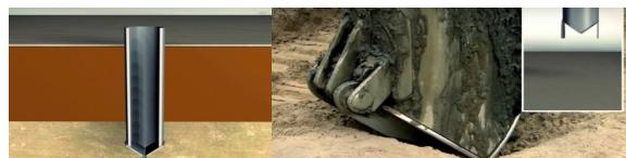
**Gambar 8.9** Pemasangan *Steel Installation Pipe*
