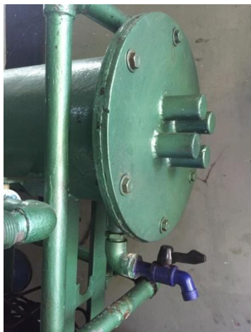
Figure 13 New drain valve installed on UV reactor
