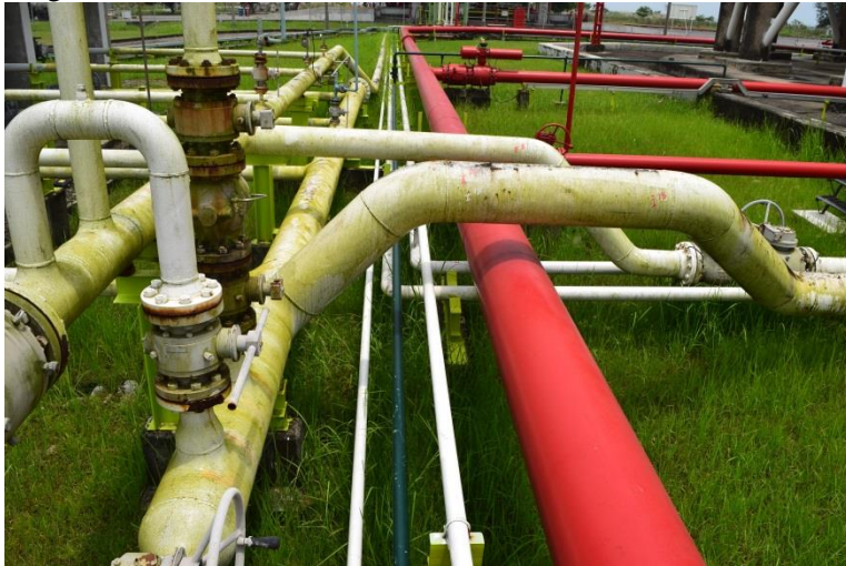
Gambar 2. 1 Pipa Header 12 Inchi
