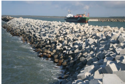
Gambar 2.7 Breakwater Kubus
