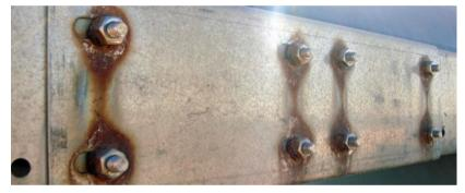
Figure 2. 6 Galvanic Corrosion (Services, n.d.)
