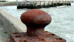
Figure 2. 5 Uniform Corrosion (International, n.d.)
