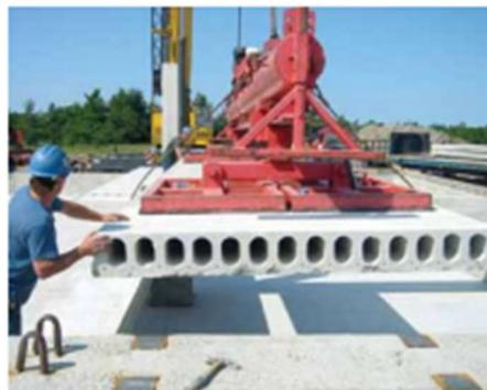
*Gambar 9 Hollow-Core Slab
