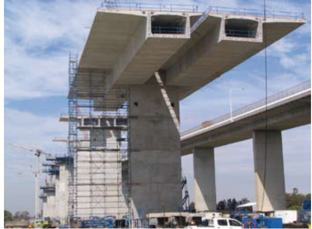
Gateway Bridge Upgrade, Brisbane, Australia
