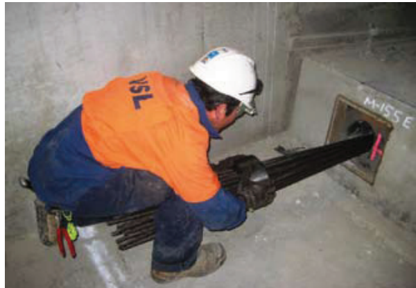
Placing of Anchor head
