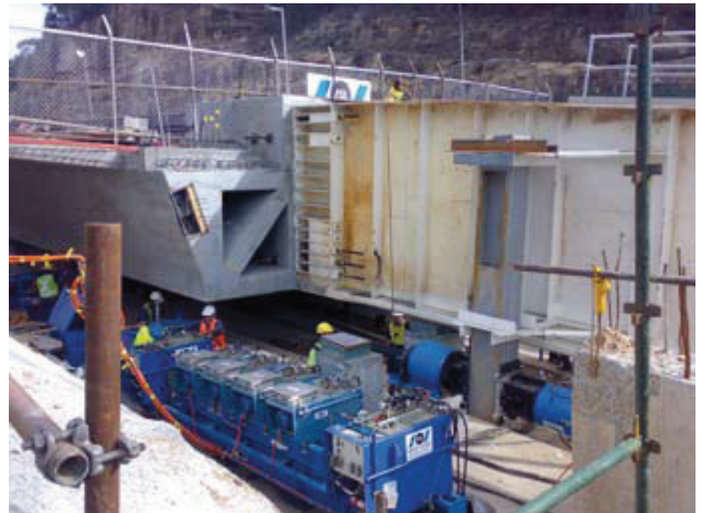
Alfords Point Bridge, Australia
