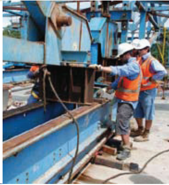
Ballina Bypass, Australia
