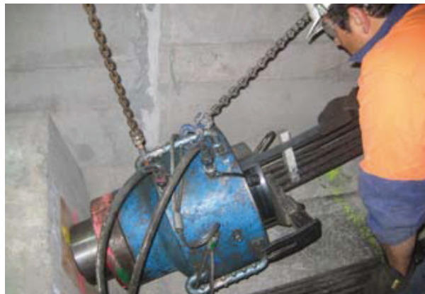
Stressing, Measuring, Seating of Wedges
