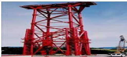
Gambar 8.10 Pemasangan Temporary Tower
