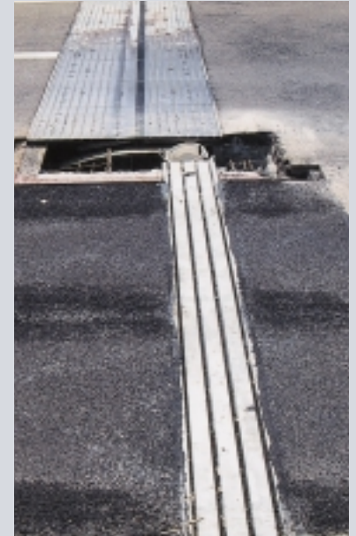
Replacement of a Roller Leaf Joint by a MAURER Swivel Joist Expansion Joint
