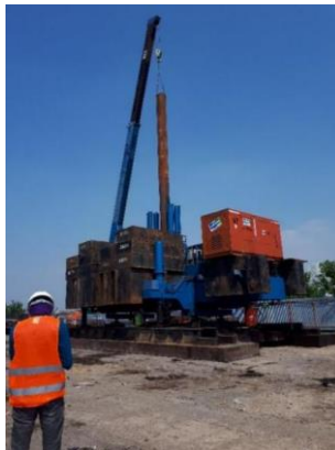
Gambar 2.1 Hydraulic Injection Pile
