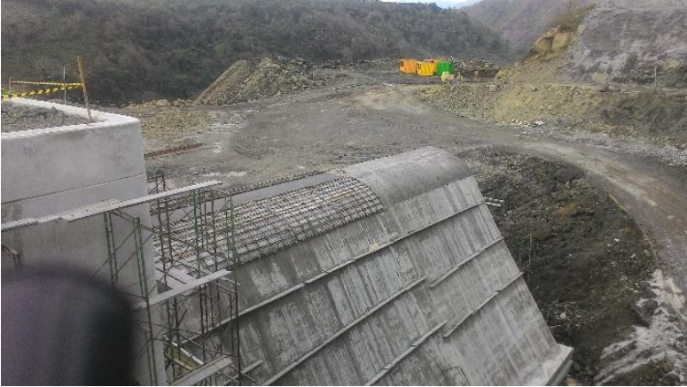
Gambar 5. Pengecoran Mercu Spillway
