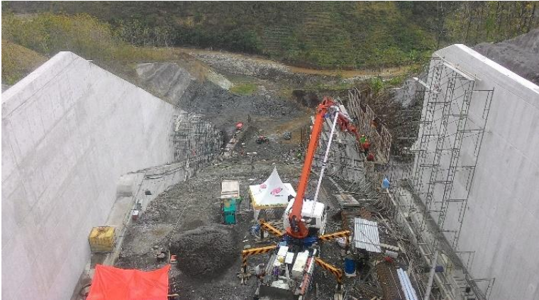
Gambar 4. Pengecoran Side Wall Spillway
