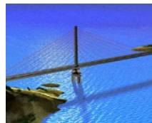
Agin Bridge (TR)
