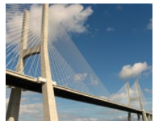
Vasco da Gama Bridge (PT)
