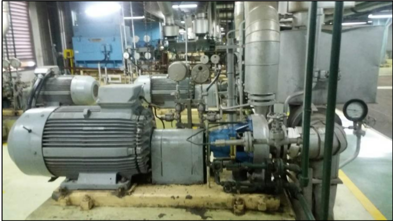
Gambar 4.9 Low Pressure Boiler Feed Pump PLTGU Blok I PT. PJB UP Gresik
