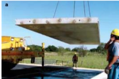
Gambar 2.2 Solid Slab (sumber: PCI 7 th Edition)
