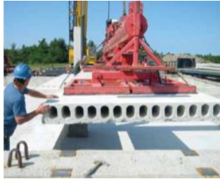
Gambar 2.1 Hollow Core Slab (sumber: PCI 7 th Edition)
