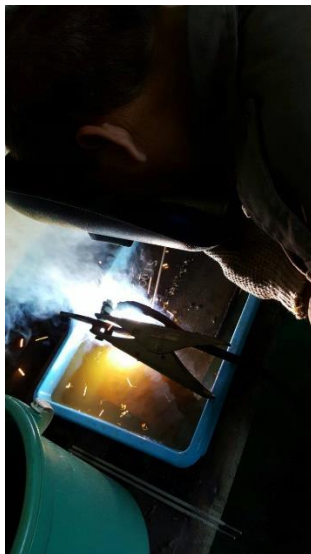
PROSES PENGELASAN UNDERWATER WELDING
