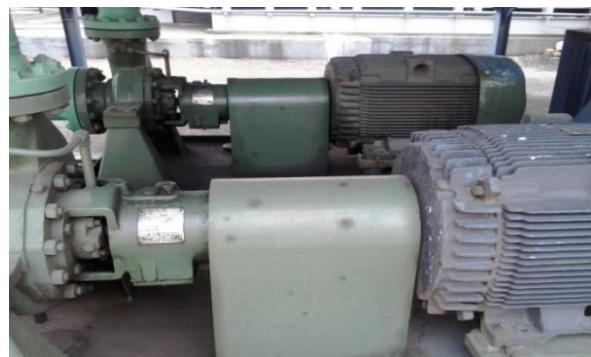
Gambar 2.3 Cooling Water Pump
