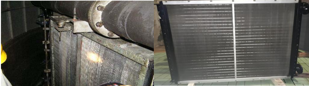
Gambar 2.17 Air cooler generator PLTA Cirata (PLTA Cirata.,1987)
