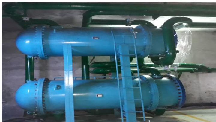
Gambar 2.20 HE antara sistem close loop PLTA Cirata (PLTA Cirata.,2009)
