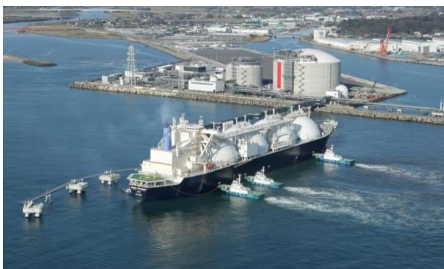
Gambar 2.5 Terminal LNG Hitachi - Jepang (Sumber: https://safety4sea.com/hitachi-lng-terminal-to-start-operations )
