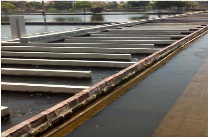
Gambar: Unit Baffled Channel
