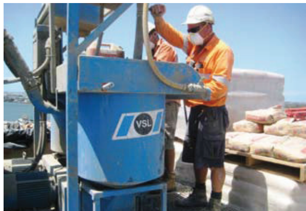
Grouting of Tendon
