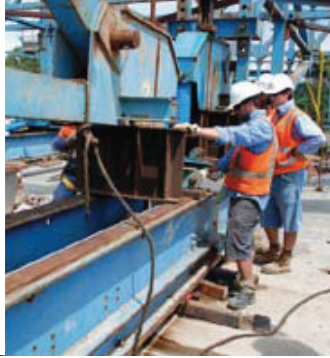
Ballina Bypass, Australia
