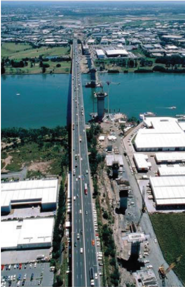
Gateway Bridge Upgrade, Brisbane, Australia
