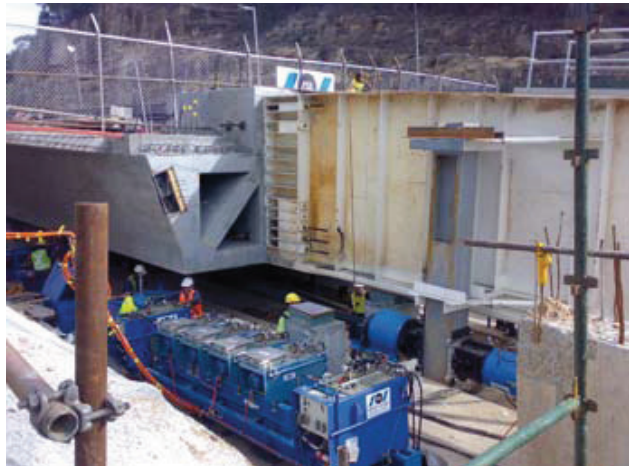
Alfords Point Bridge, Australia
